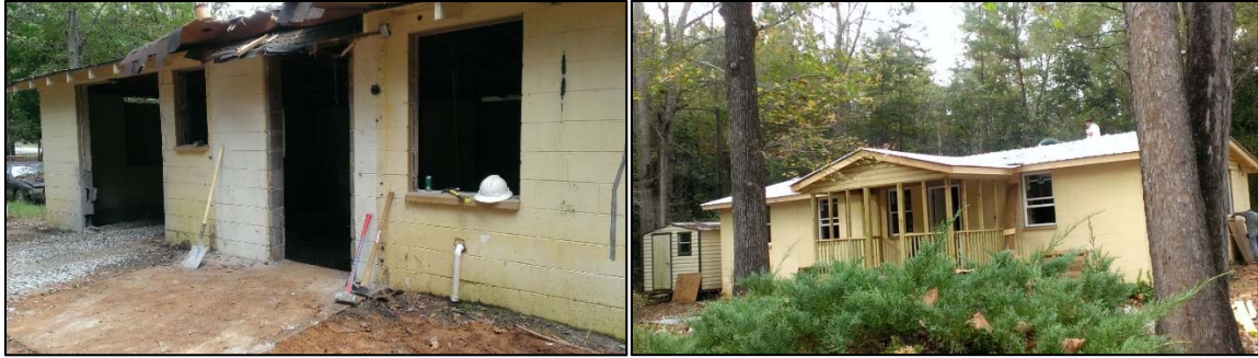
Housing Reconstruction Project - Before and After
