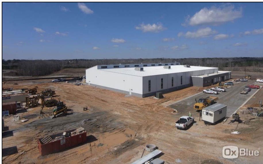
Construction of Schmidt Automotive USA, L.P. Facility in Auburn
