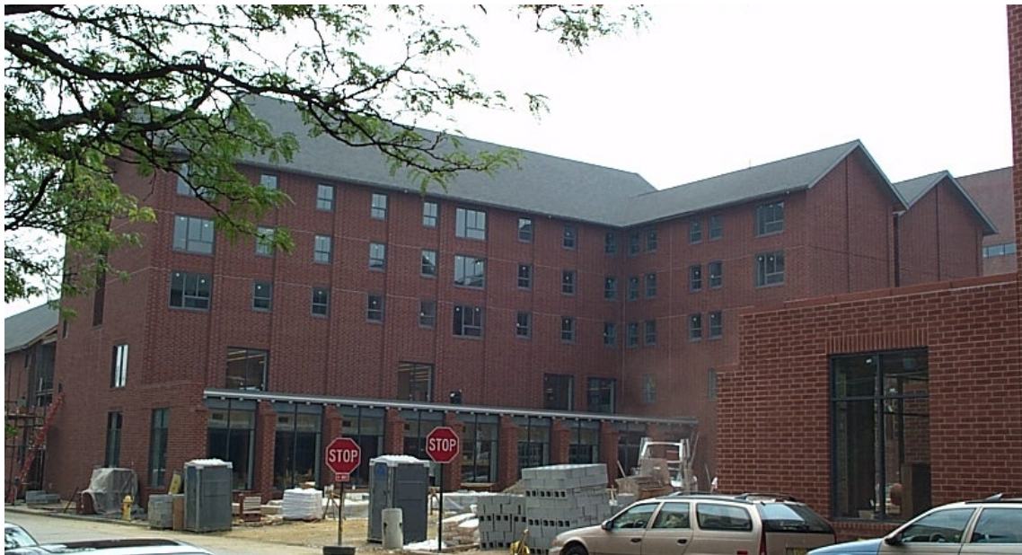
Figure 2: The façade of Building C near its completion
