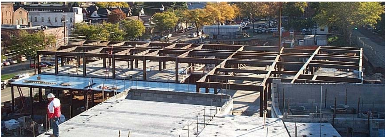
Figure 6: Building C – The steel frame as seen from the west face.
